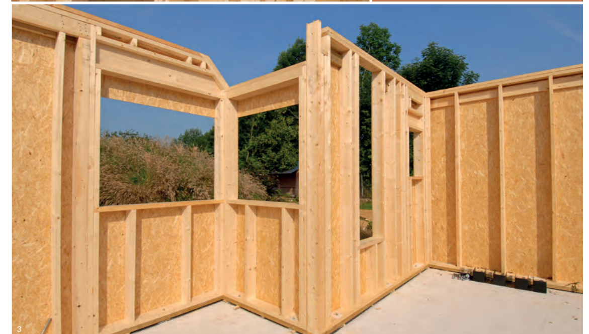
1, 2 and 3. Vertical uprights and horizontal rails for timber-framed walls
