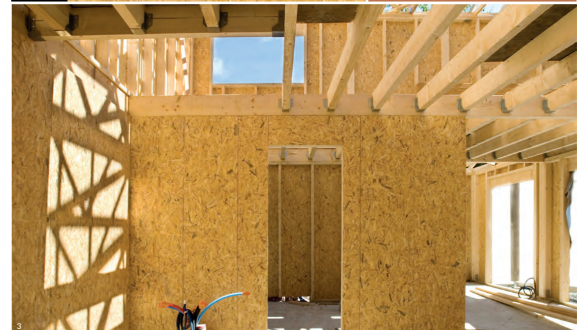
1, 2 and 3. Backing board panels for timber-framed walls
