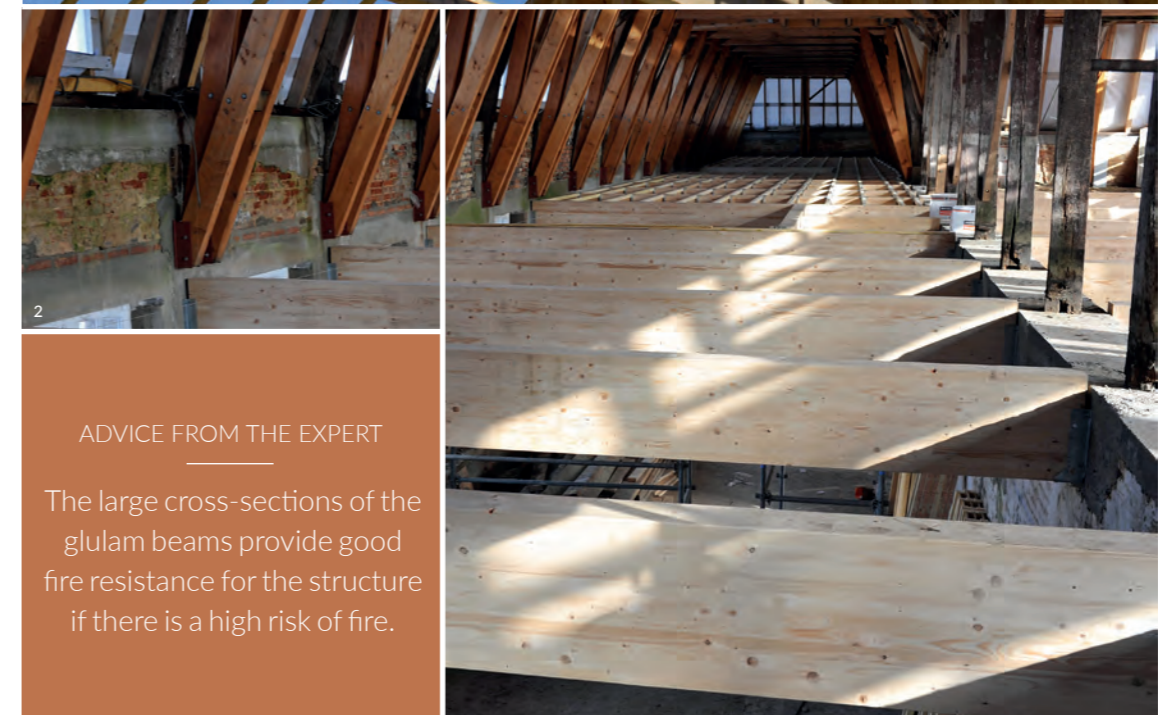
1. Long-span purlins/2. Load-bearing floor beams
