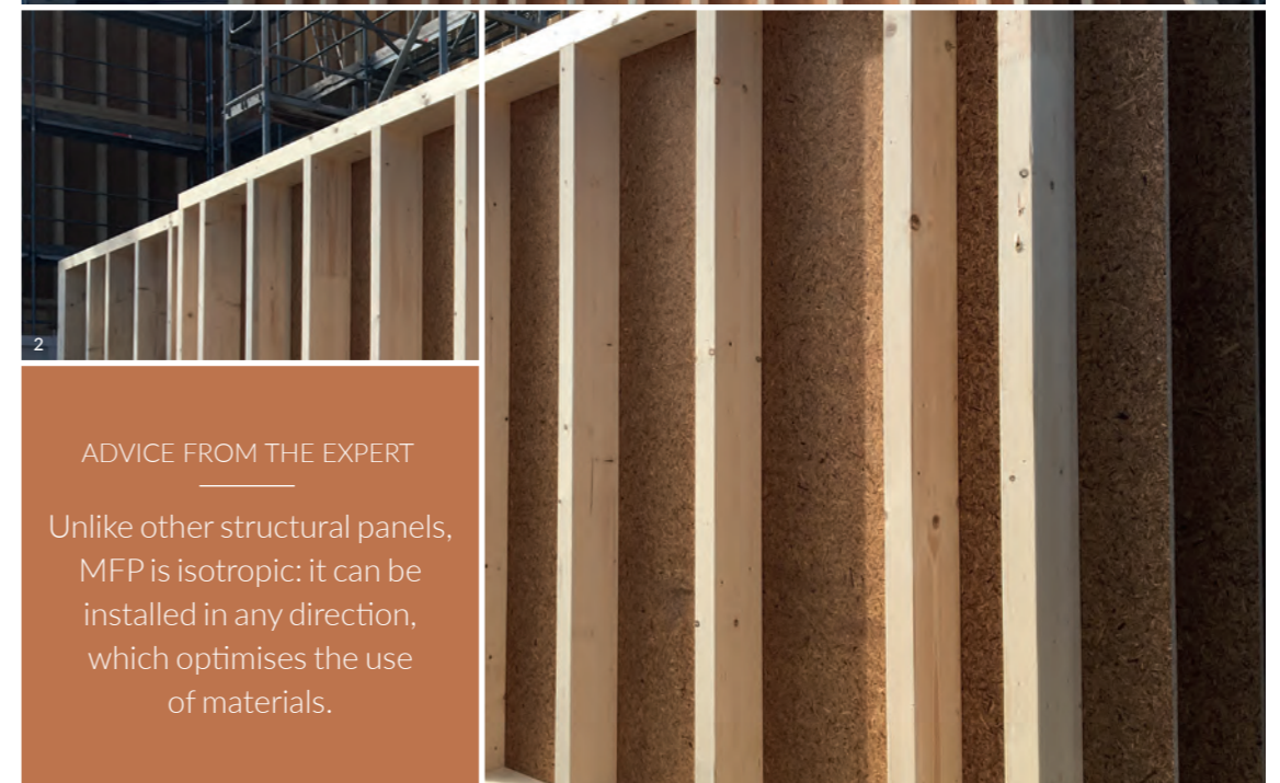
1 and 2 Backing board panels for timber-framed walls
